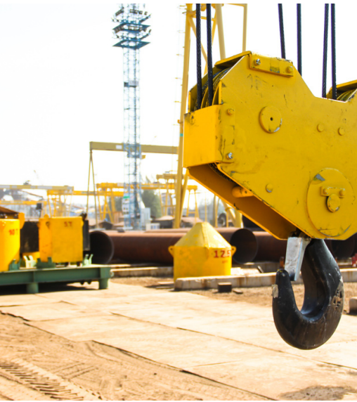
Pile Load Test
