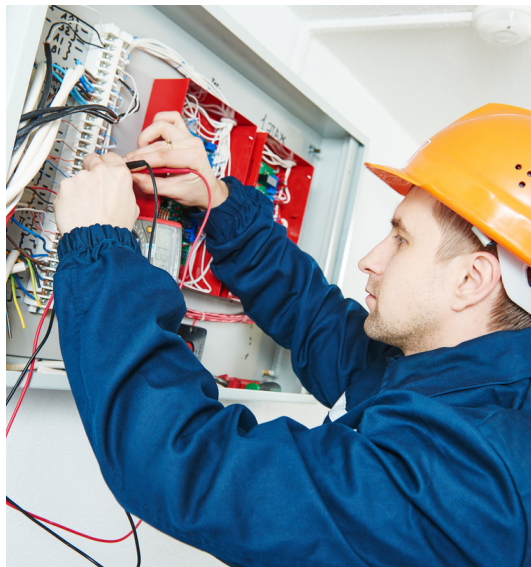
Electrical Resistivity Test
